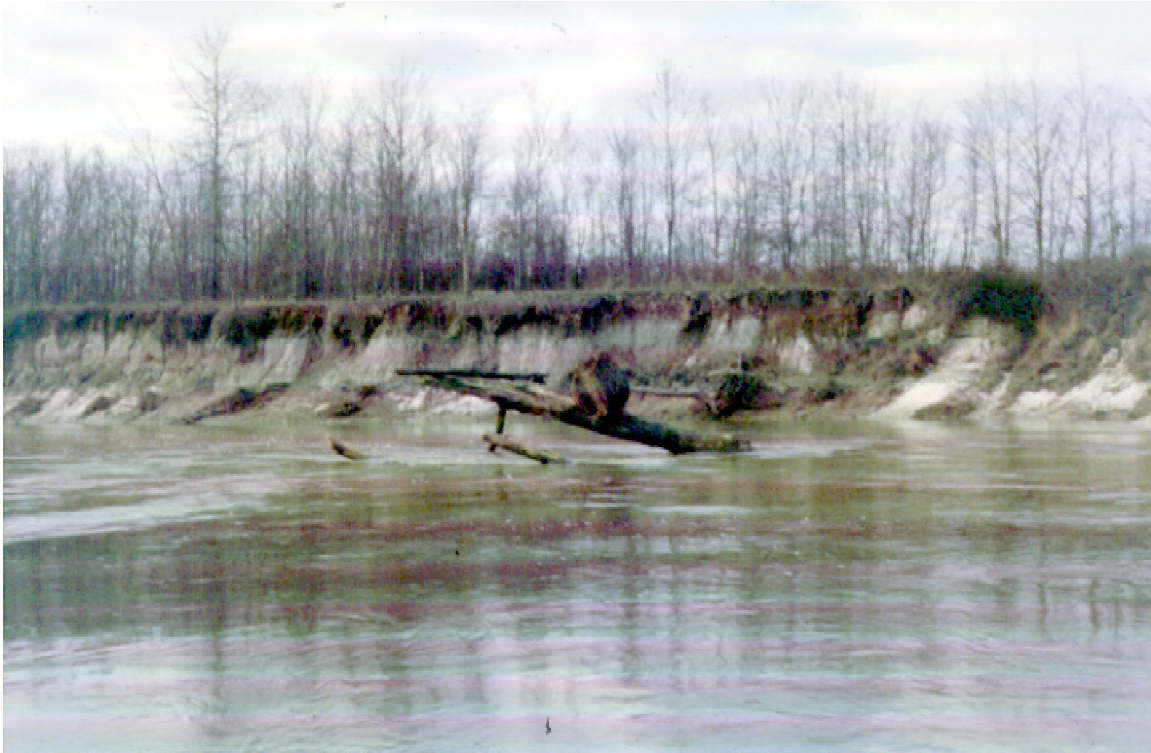
Figure 1. Headcutting on the Wolf River, Tennessee
