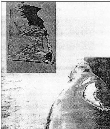
Figure 1. Geotextile tube deployed in field, with S. alterniflora to right and open water to left; inset shows dredged material island with geotextile tubes
